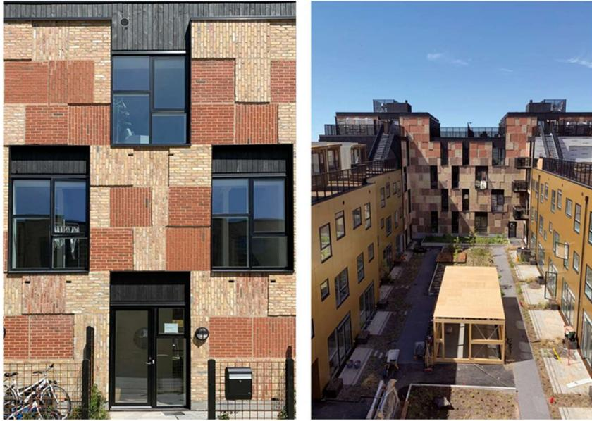
*Figure 4-2. The Resource Rows project incorporates recycled brickwork panels, composed of cut-out segments from old brick walls, creating a colorful patchwork with a knitted texture.*
