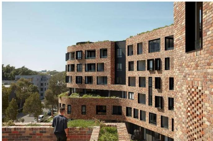
*Figure 4-4. Arkadia is made from recycled bricks that have been formed so that they create solar shading to the north and west with windows that allow cross ventilation while avoiding full summer sun penetration.*
