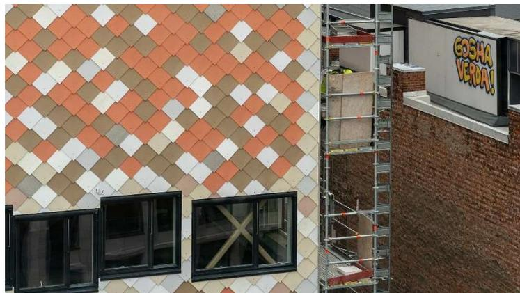
*Figure 4-6. The façade panels used in the Kristian August Gate 13 project were sourced from a 35-year-old housing association building in Trondheim. The panels were carefully cut and adapted to match the dimensions needed for the project, resulting in 3,819 processed panels being delivered.*
