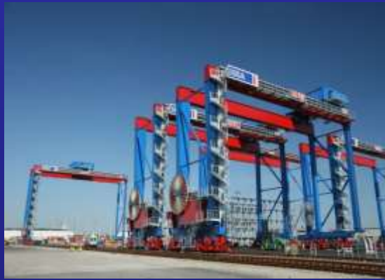
Unmanned container handling
