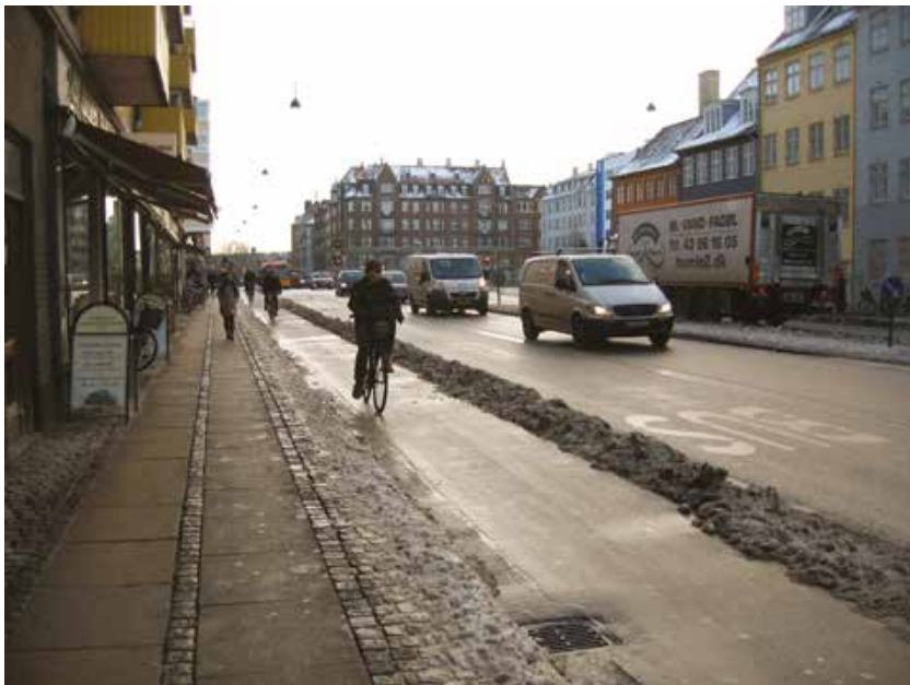
Fig. 24. In Copenhagen, planners have added a half-metre wide space for snow between the cycle path and road, eliminating the need to transport snow during a normal winter.
