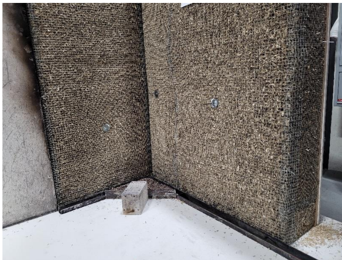
A close up of the vertical outer edge of the long wing in test 3.
