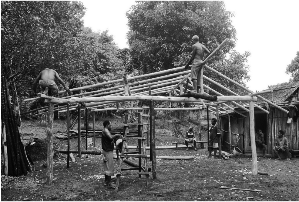
Photo 5: Men help their relative to build a house
