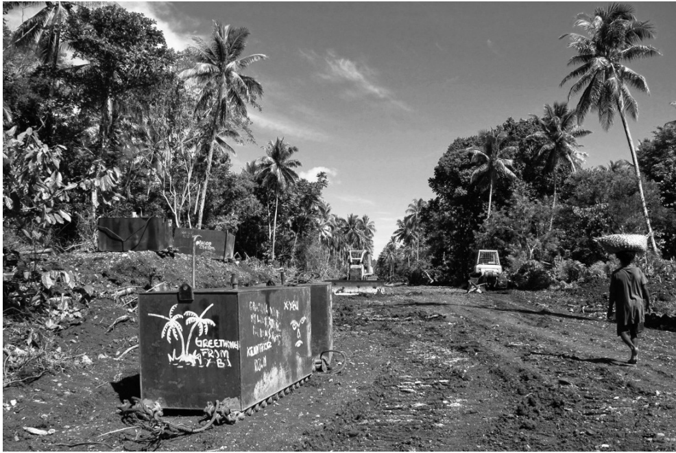
Photo 15: Newly widened logging road in Wide Bay
